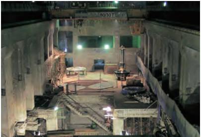
Powerhouse at Musi Project, Indonesia
