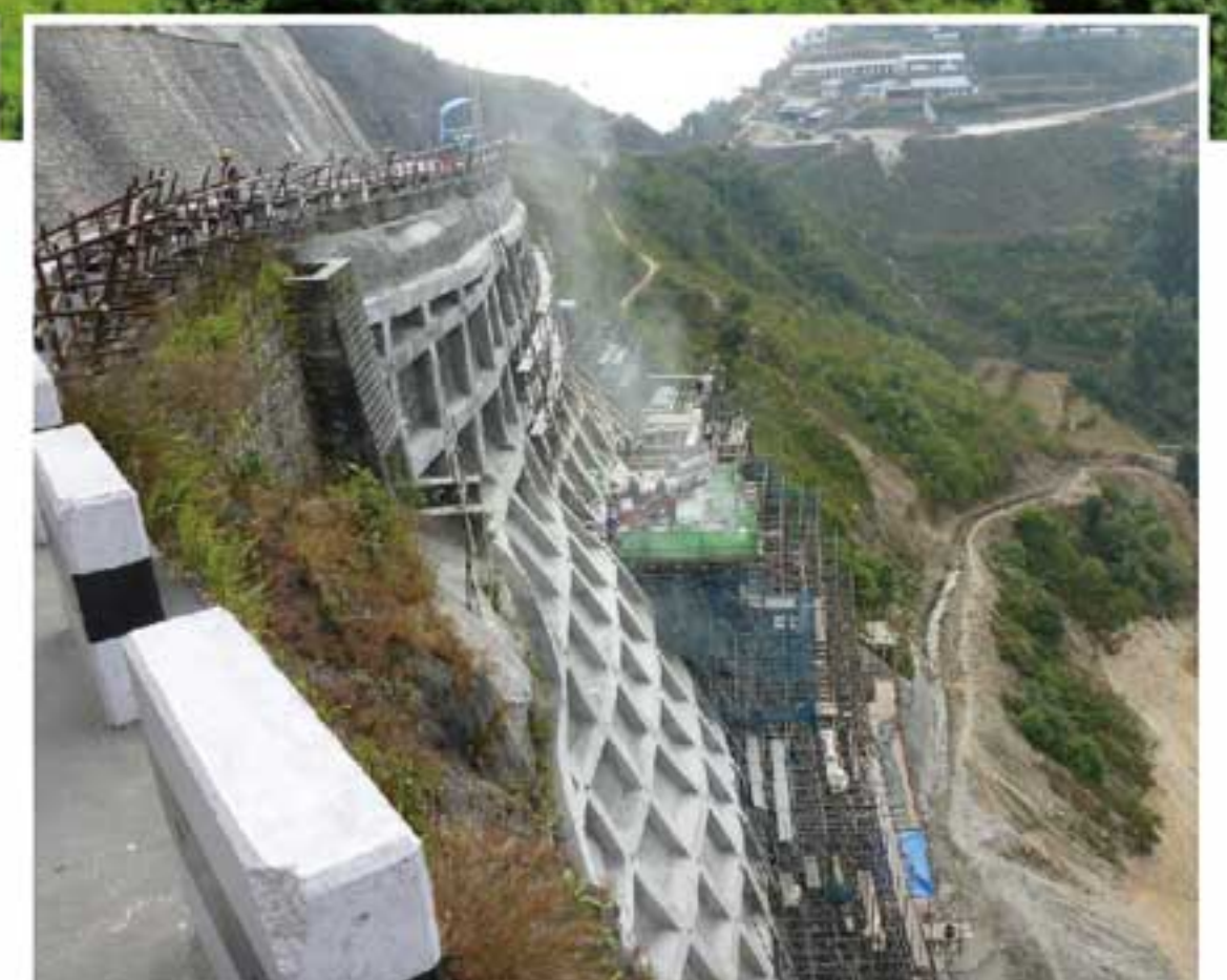
Ground anchor works
