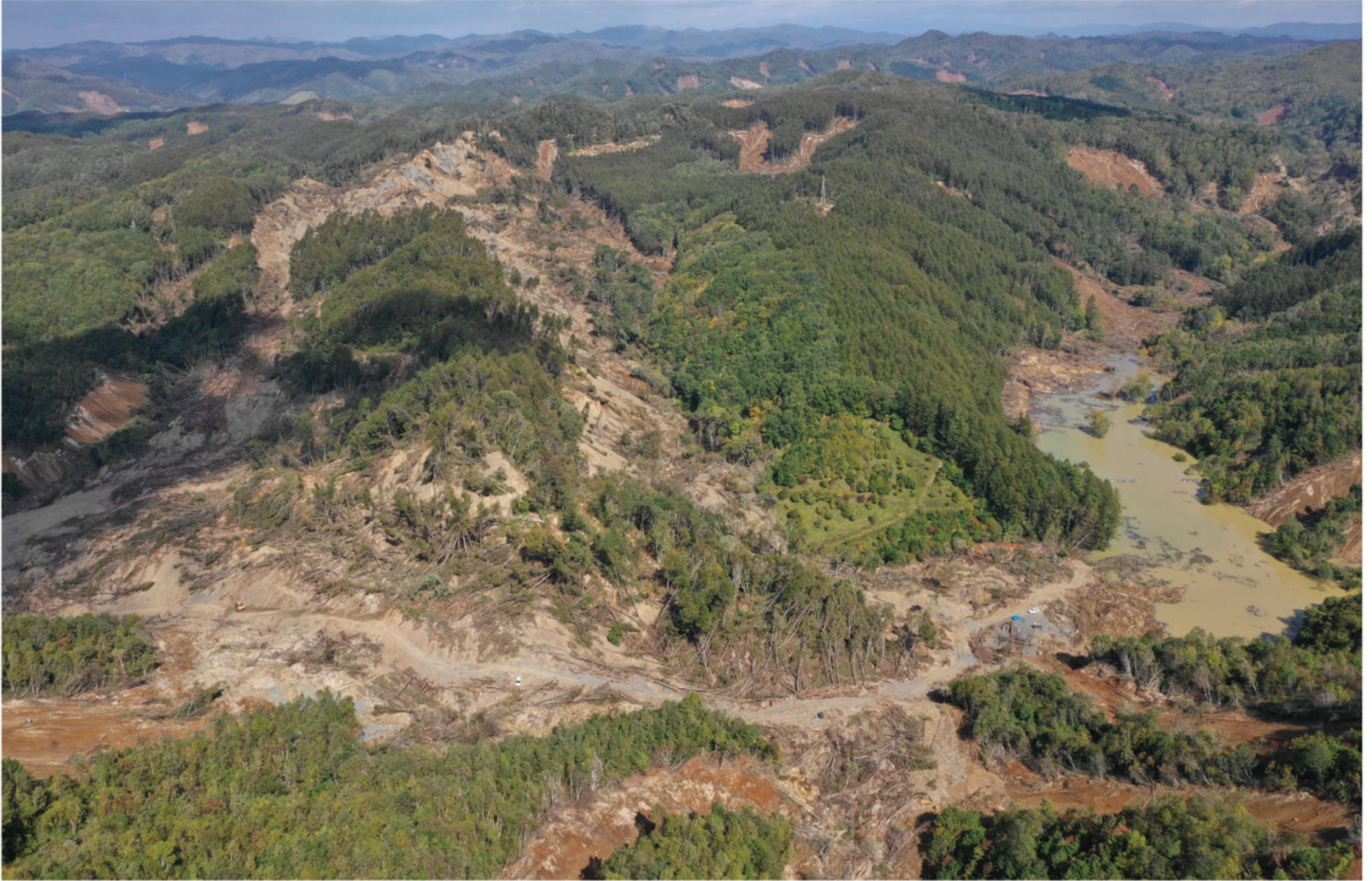
Nippon Koei immediately surveyed the landslide dam formed due to slope failures following the 2018 Hokkaido Eastern Iburu Earthquake, and thereby proposed emergency and permanent measures, contributing to minimizing the damage (Photo: Hokkaido Regional Development Bureau, Ministry of Land, Infrastructure, Transport and Tourism)
