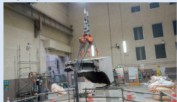
Removing a concrete section cut using a wire saw
