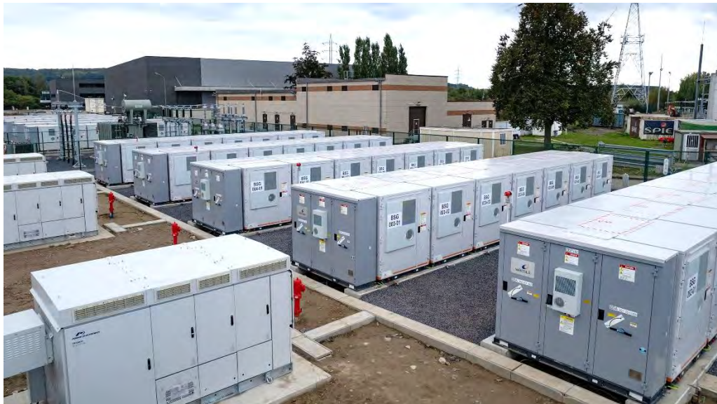
■ View of Ruien's 25 MW/100 MWh storage location (about 0.5 ha)
