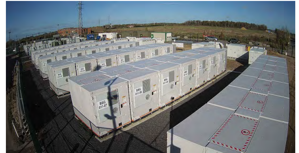
Construction site of Ruien power storage station
