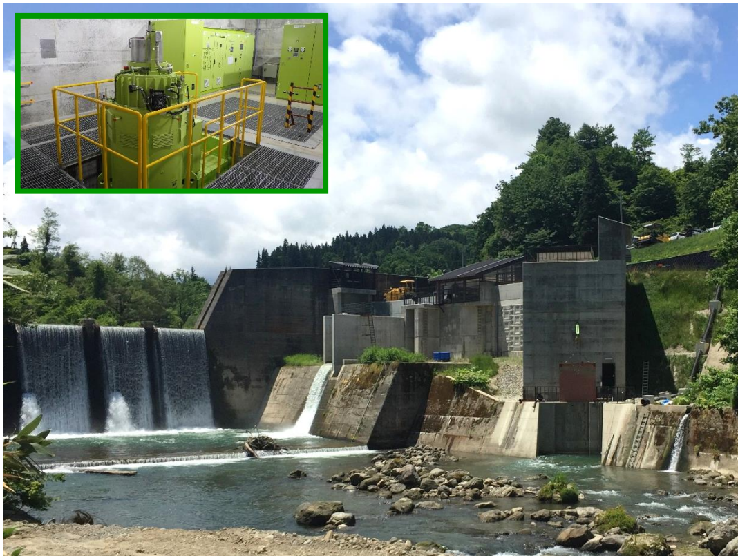
Ohkura Masudama Hydroelectric Power Plant
