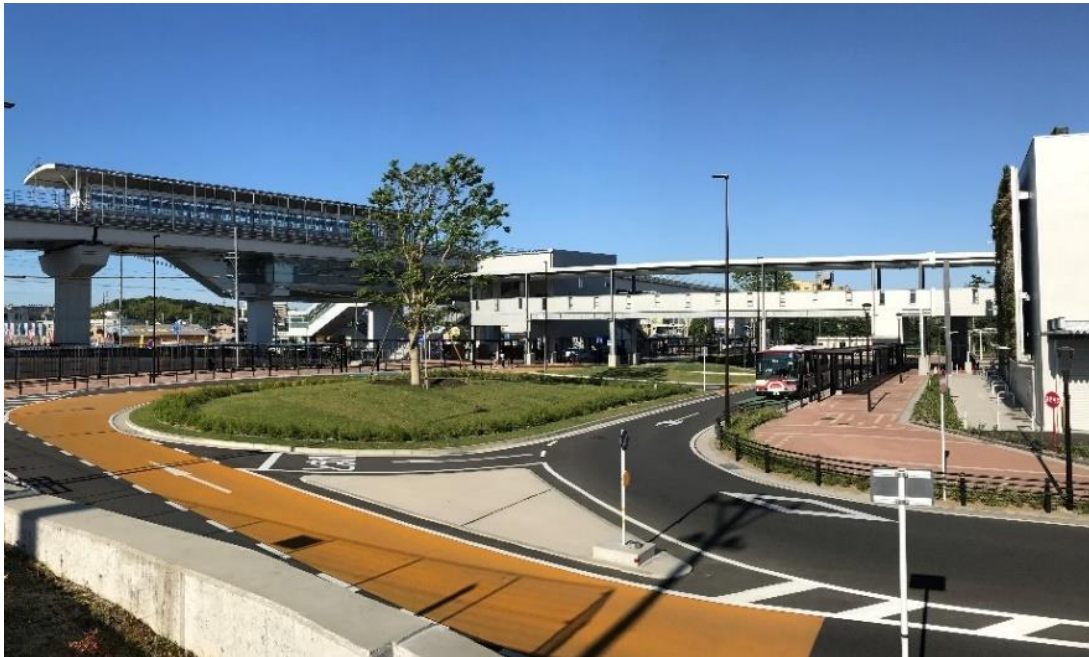
Nagakute central land readjustment project: Linimo Nagakute Kosenjo Station plaza
