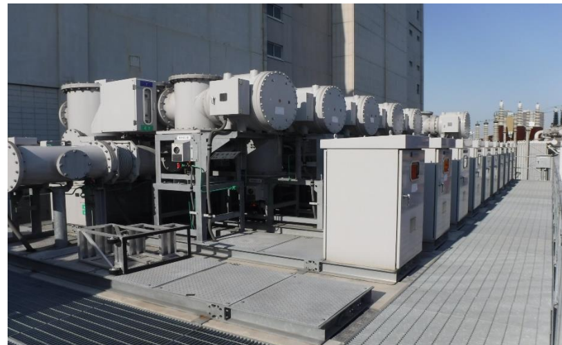
Gas insulated switchgear
