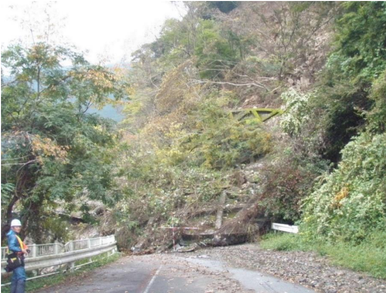
Urayama Dam road disaster
