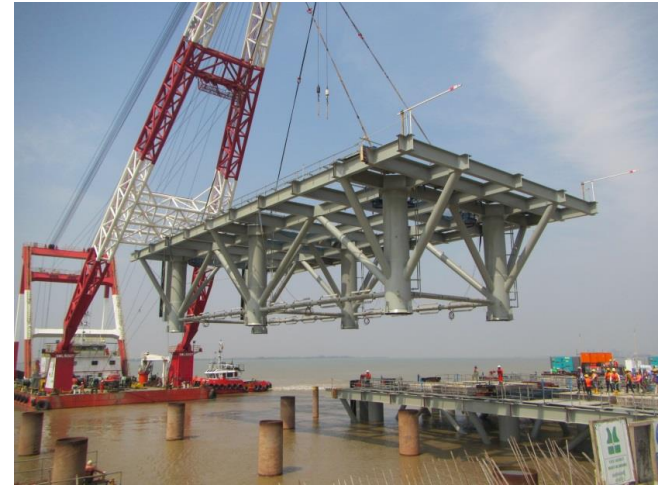
Installation of the jacket (250t)
