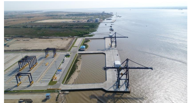
Multi-purpose terminal wharf and Yangon River
