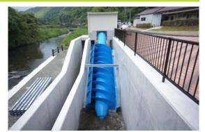
\*The photo shows a demonstration experiment at the Kotaka power plant (the Kotaka weir screw turbine demonstration facilities)
