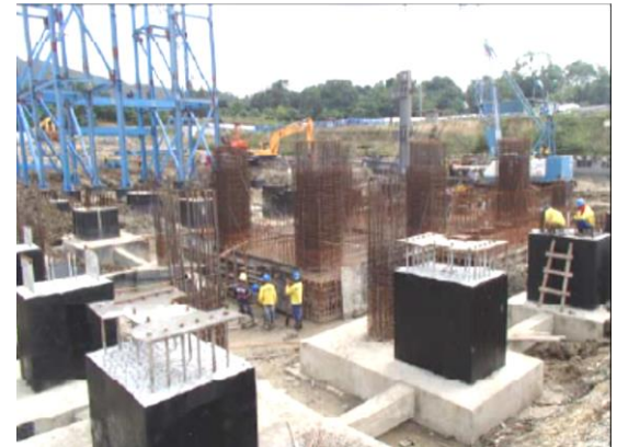
Foundation of the building of a turbine and electric generator
