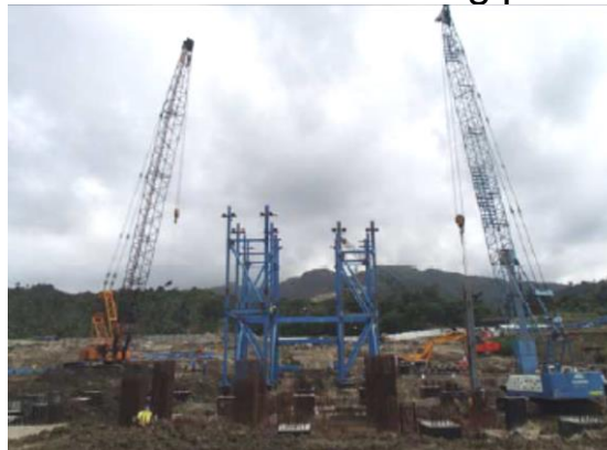
Construction of boiler steel frames
