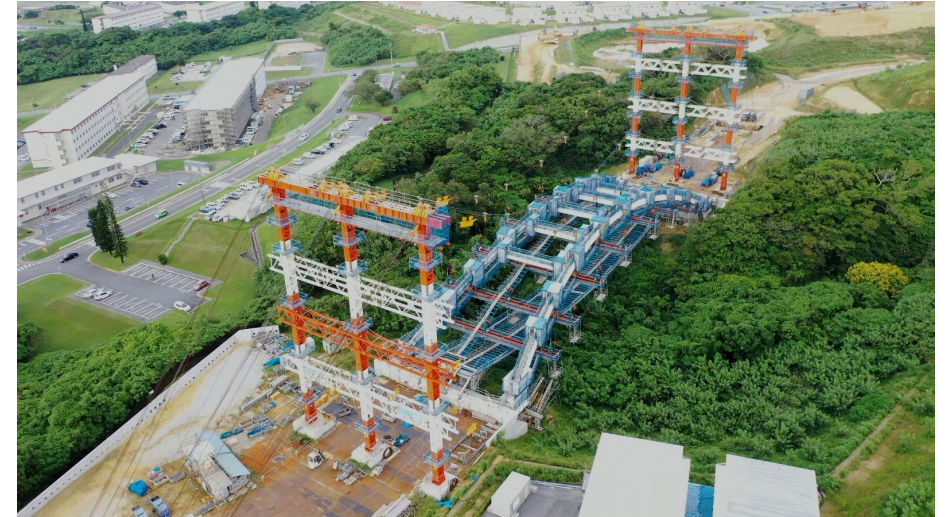
Current state of the Nishi Futenma Bridge(provisional name)
