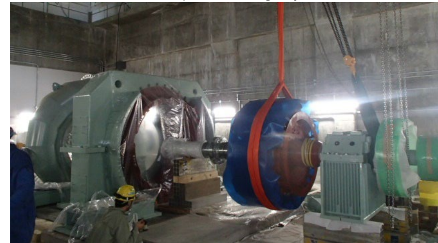
Insertion of a generator rotor
