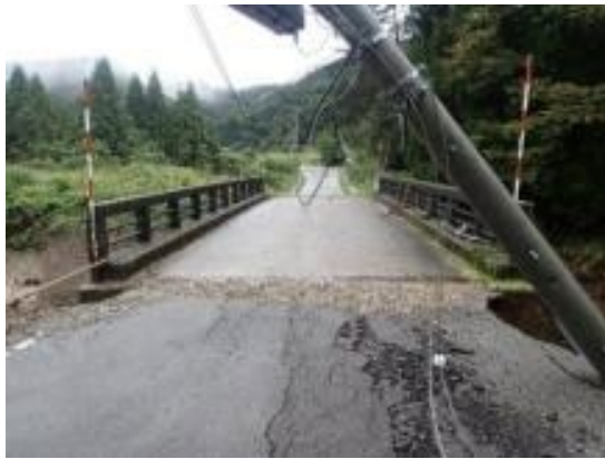
Munesue Bridge damaged by the September downpours
