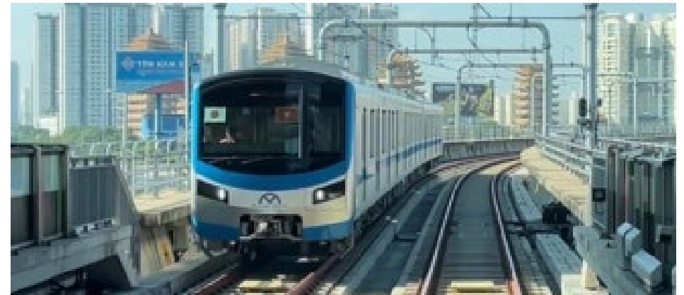
A train on Line 1 in operation
