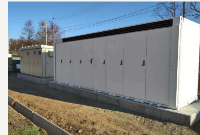
Battery Storage and Energy Management System
