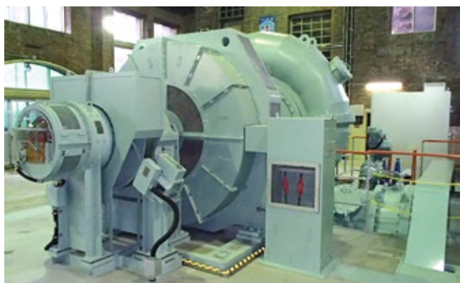
Horizontal synchronous generator
