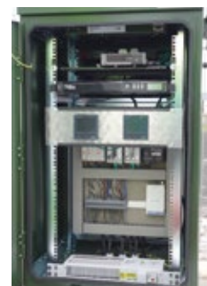
Storage battery control system
