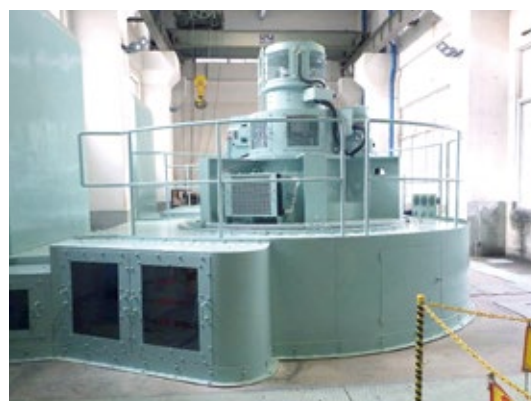
Vertical synchronous generator
