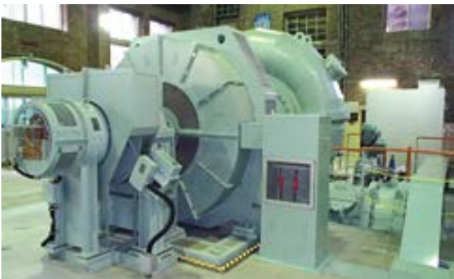
Horizontal synchronous generator
