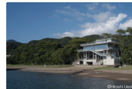
Tsunami evacuation complex Terrasse Orange toi
