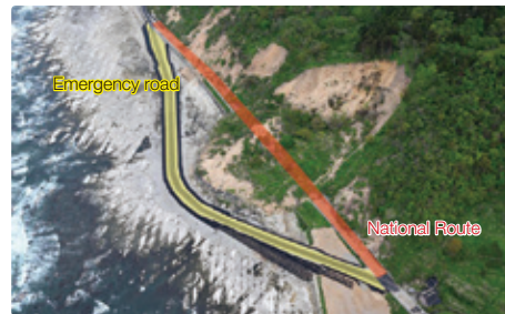
National Route 249 after emergency repairs
