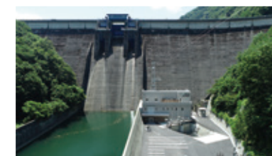
Miwa Dam and Miwa Power Plant
