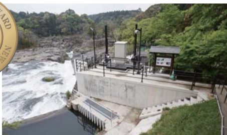
Shinsogi Micro Hydropower Plant
