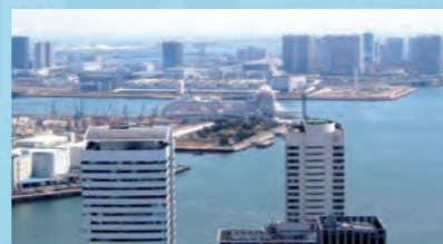
Tokyo Coastal Highway Construction Project
