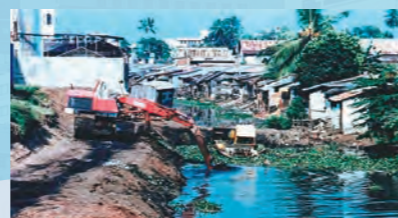
Sri Lanka Greater Colombo Flood Control and Environment Improvement Project
