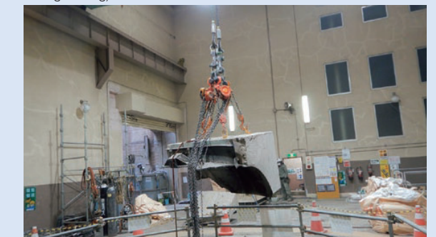
Removing a concrete section cut using a wire saw
